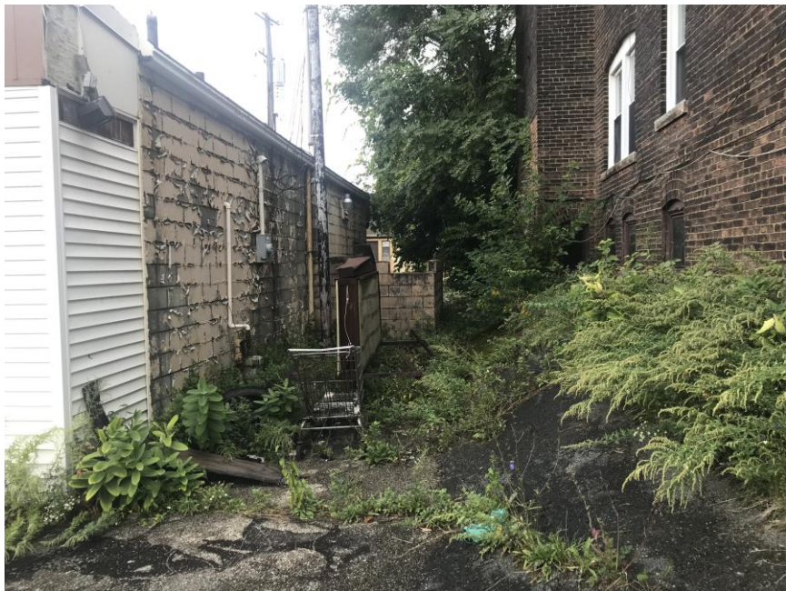
Photo 3 – A view of rear of the building and adjoining apartment building.
