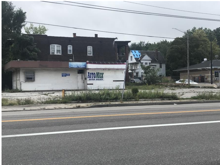
Photo 1 – A view of the Property looking across Euclid Avenue.
