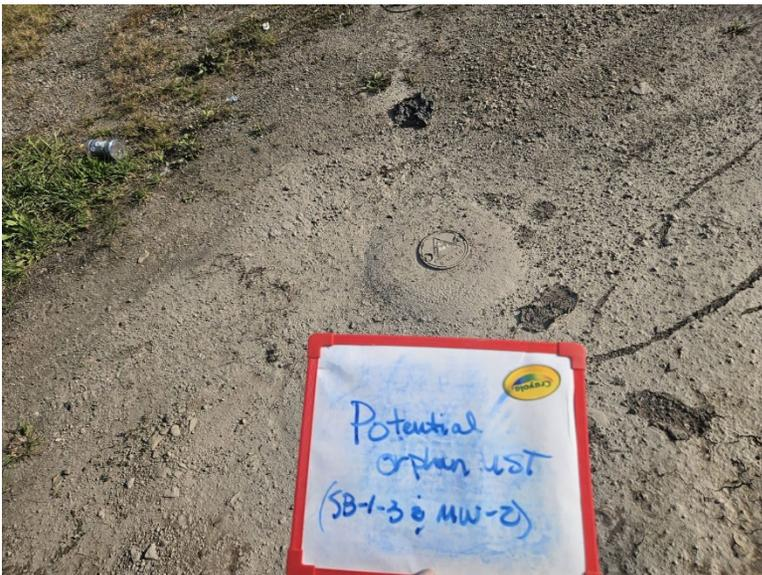
Photo 15: View of monitoring well proximate to potential orphan UST.
